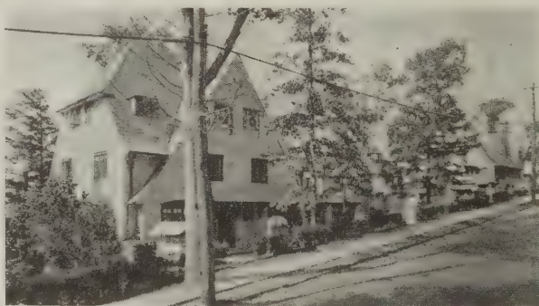
VIEW LOOKING NORTH, OAK COURT TERRACE DEVELOPMENT
